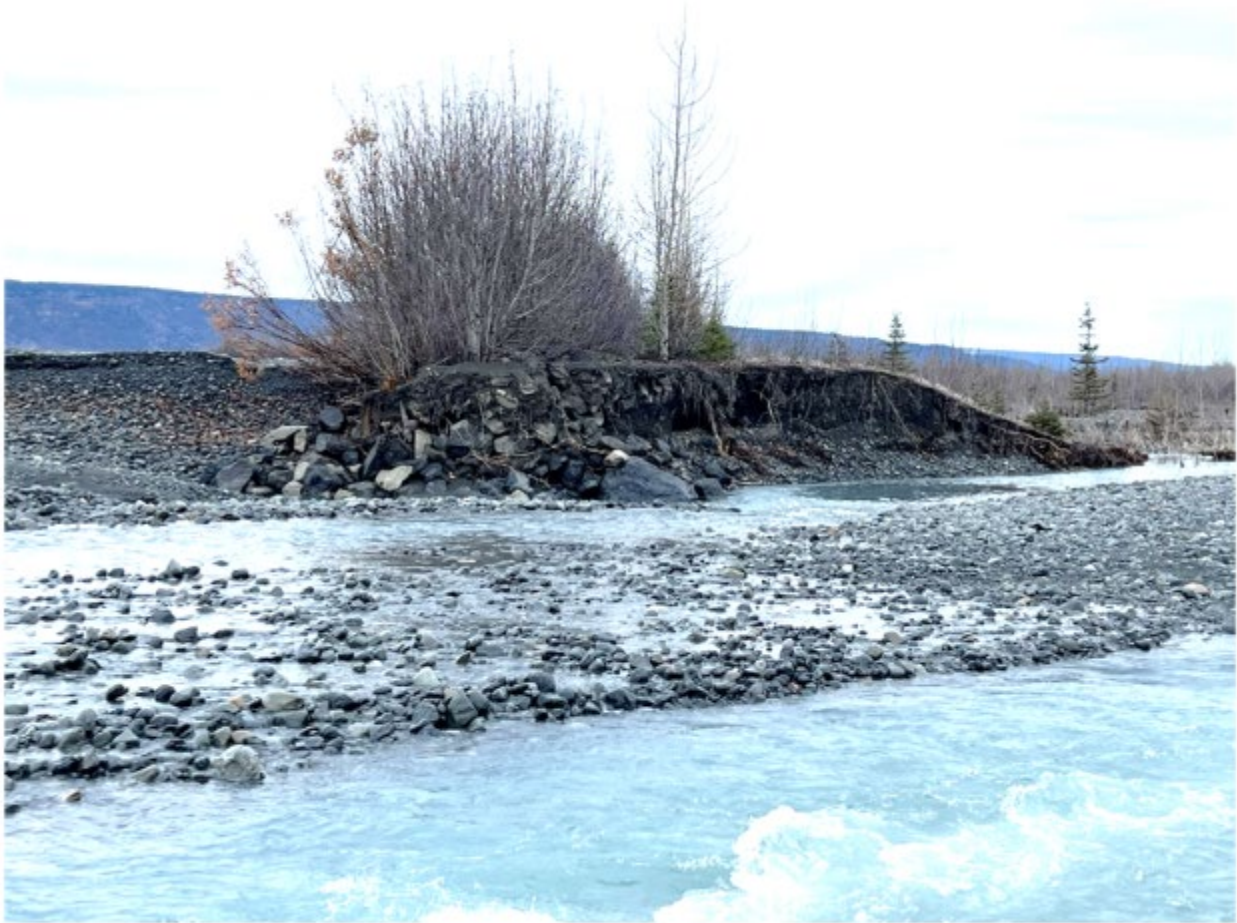
Photo 5-3 Cross section of levee at breach location, November 2, 2023.
